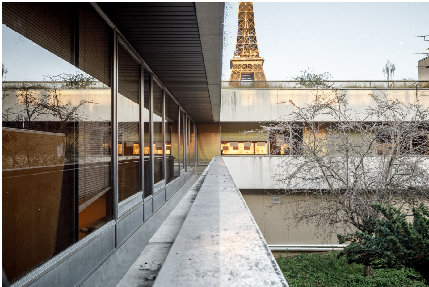
Photographie du centre Emile Anthoine avant travaux, prise depuis le cœur d'îlot, 2022 | © 11h45 Photograph of the Emile Anthoine center before renovation, taken from the inner court of the block, 2022 | © 11h45
